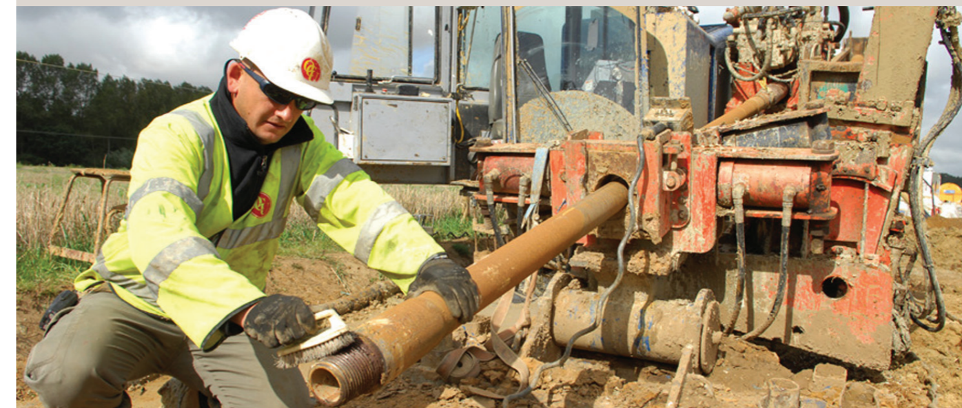
A horizontal drilling technique will be used at key locations along the cable route to minimise disruption
